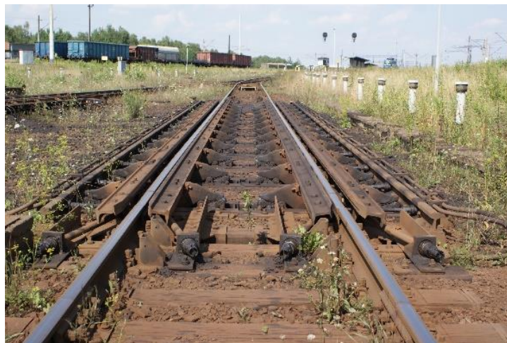
Figure 2. Marshalling yard Tarnowskie Góry, voivodeship Silesian, Poland – rail brake / technical and exploitation device
